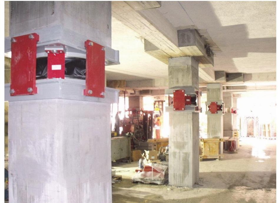
Installation of the isolation unit at the top of first basement columns (Freysaş Inc.)
